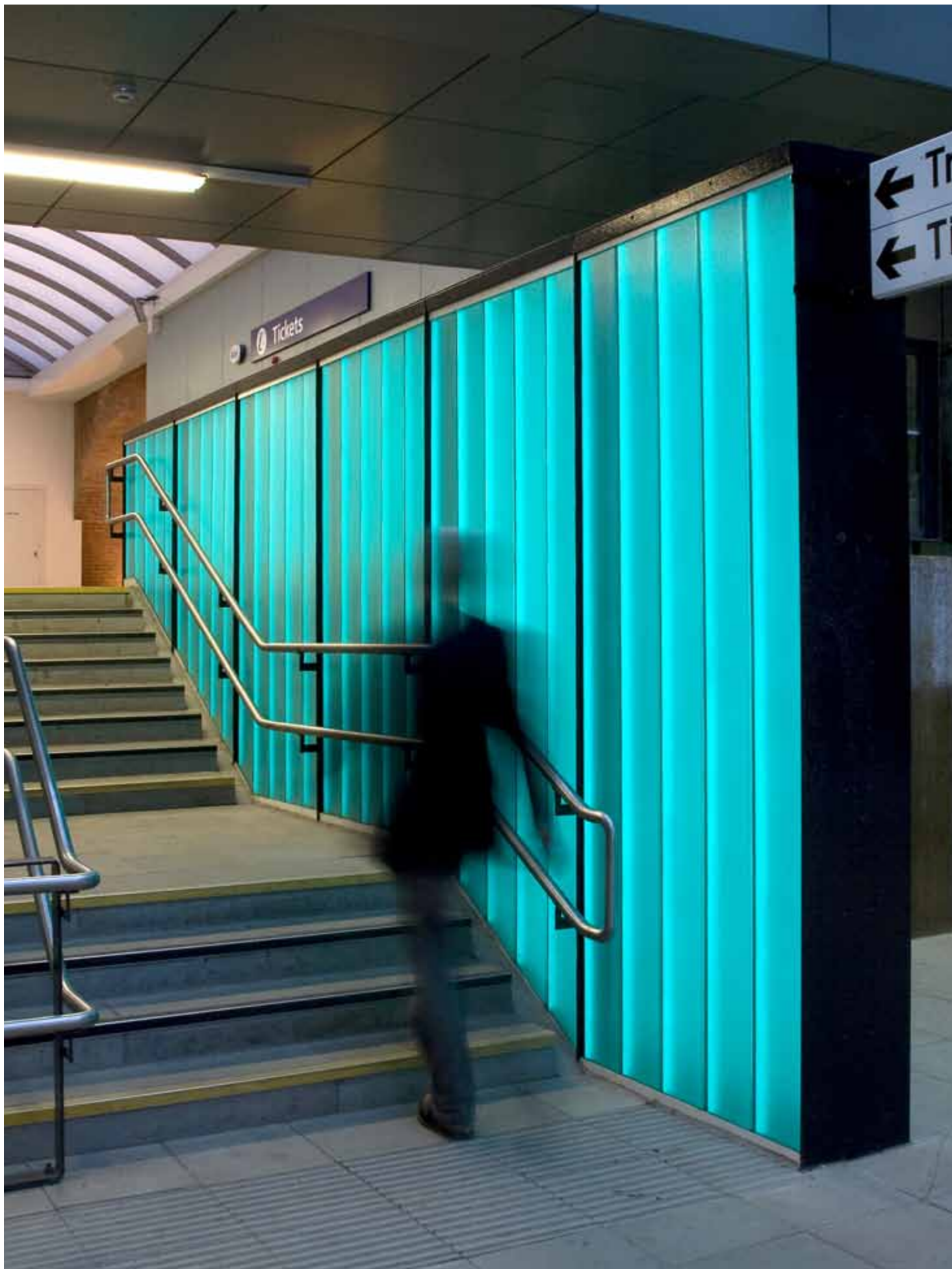
Project – Salford Station Architect – Austin-Smith:Lord Main Contractor – J.Murphy + Sons Ltd Photography – Simon Warren Glass – (K22/60/7) SP2 S/B Cast Toughened Light – DFL - 0175- G Inverter – 12 KND X2 Control – On/Off
